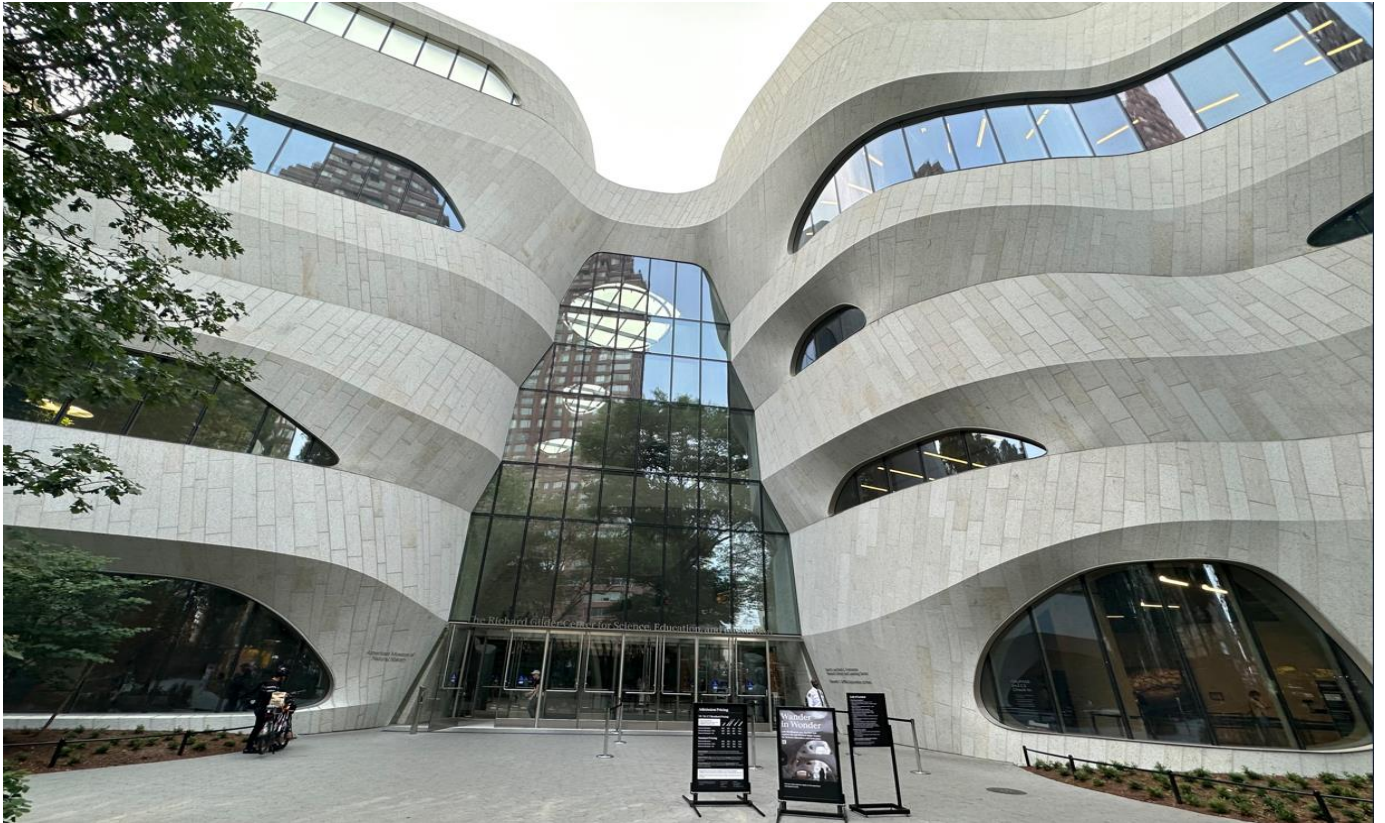
Facade focusing on organic curves
